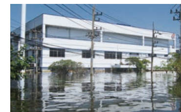
Medical factory inundated with 3 meters of water
