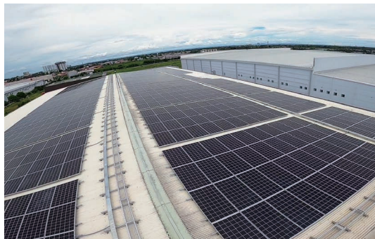
Installing solar panels at Cebu Factory
