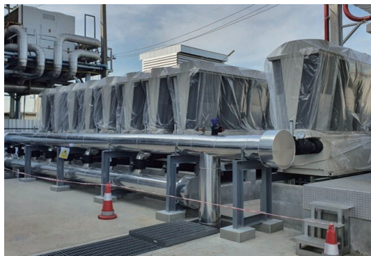
Installing energy-saving chillers
