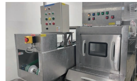
Installing cafeteria equipment such as water-saving dishwashers
